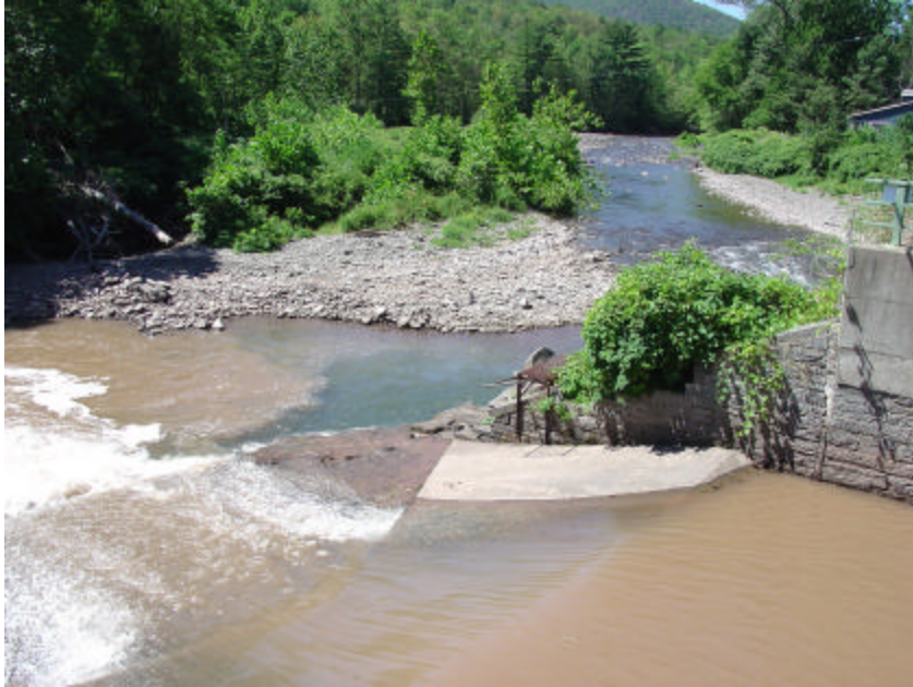
Figure 2.5. Transference of turbid water from the Schoharie basin to the Esopus Creek via the Shandaken Tunnel.
