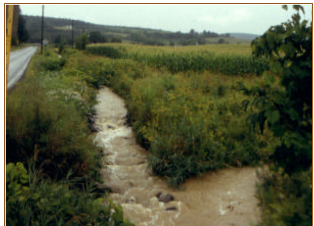
Figure 2.12 roadside ditch transporting water and sediment material downstream
