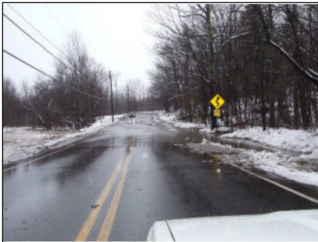
Figure 2.11 Flooding along State Route 296, Town of Windham
