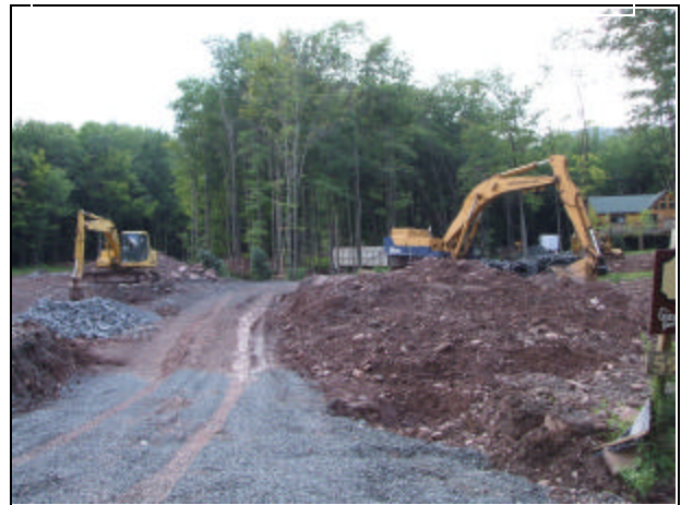
Figure 2.15 Construction of a private road in a major subdivision, Hunter
